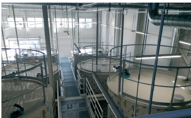
PP container for process water
